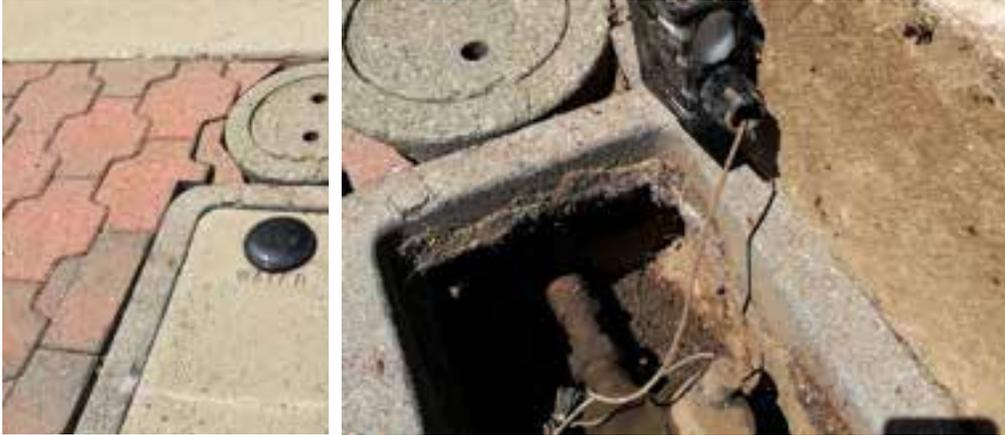
*Figure 3: NB-IoT Water Meter Curbside Installation.*
