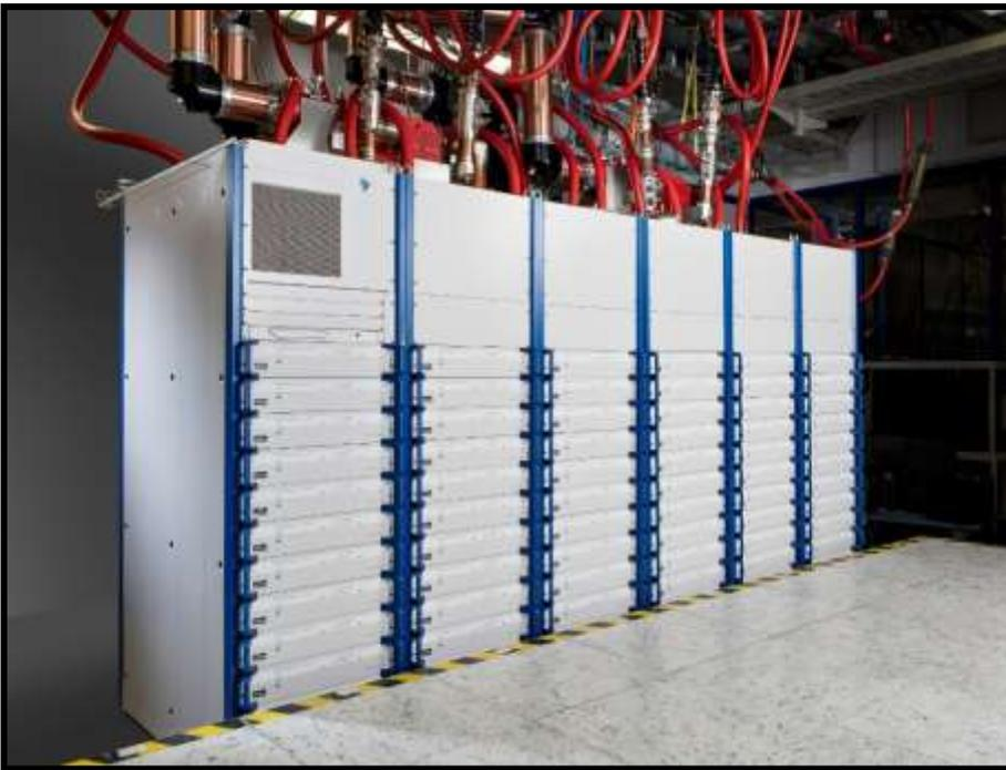
**Figure 2: R&S THU9evo with 106kW TPO (ATSC).**
