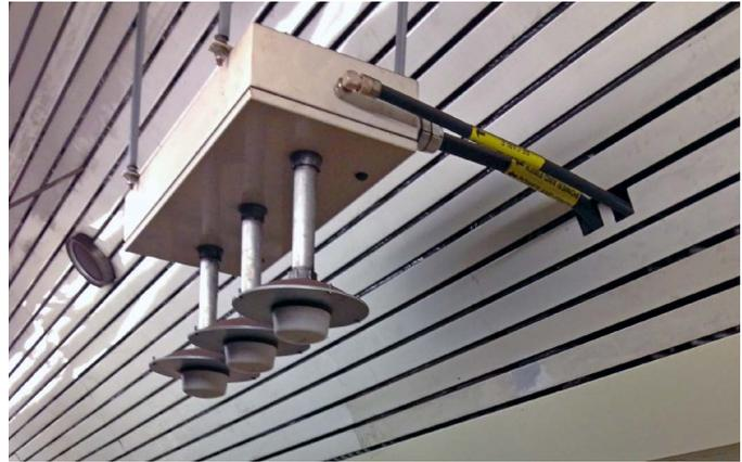
DAS with RF access point and antennas in the Fifth Ave. / 53rd Street station. Additional antennas are mounted on the back side of the wall. (Courtesy of Wikimedia Commons)
