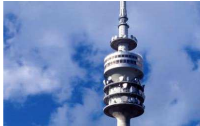
Operators of wireless communications and broadcast networks
